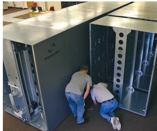
Figure 4 Construction of the Sun SL8500 ATLs.
